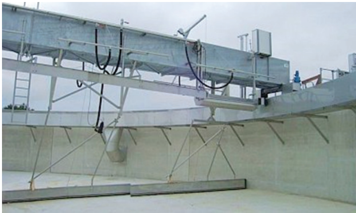
Figure 5.6 Scraper arms move the settled solids to the center of the tank [16]
