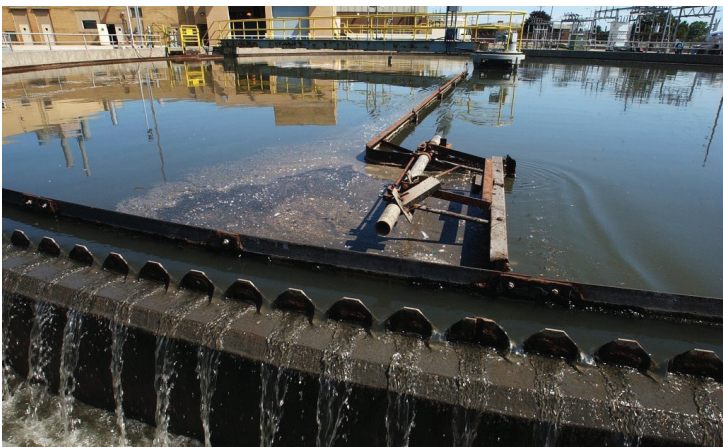
Figure 5.7 Circular sedimentation tank showing grease skimmer and effluent weirs
