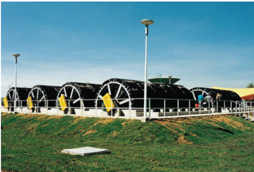
Figure 6.8 Rotating biological contractor
