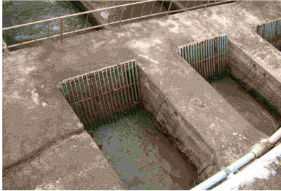
Figure 4.2 Coarse screens [3]
